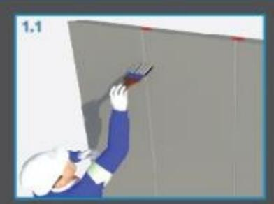
Clean the surface to be free from dust, grease and other contaminants, in case the gap is deep and wide, can install backing rod first.
