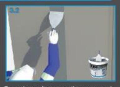
To make surface smoother, can apply second layer of RHINOZ Hybrid Jointing Compound after 2-3 hours
