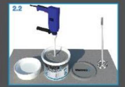
Mix thoroughly using spinning mixer at low speed of 300-500 rpm, until become homogeneous.
